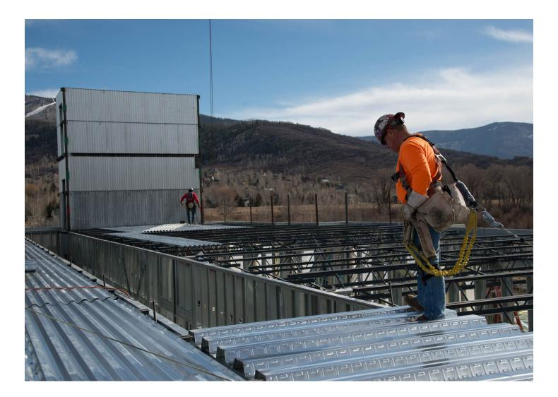
**66** The overall composite design eliminates shoring and allows for open spans, all while using a thinner slab. That saves head room and makes clients happier."
