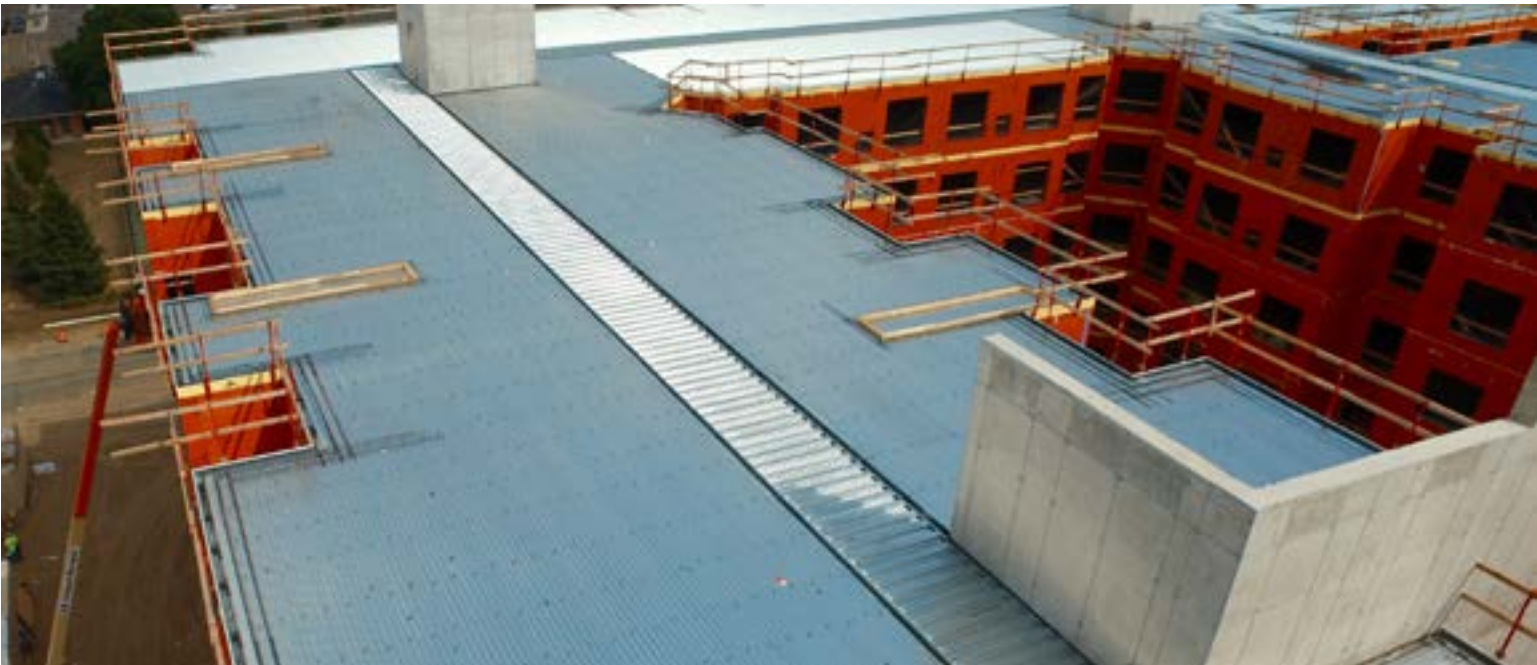
Ecospan® joists span from the corridor wall to the building exterior. Photo courtesy Rick Gilchrist Co., Inc.
