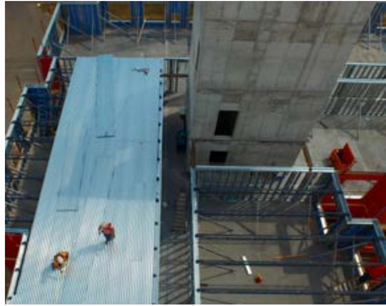
Ecospan® is installed quickly and easily, with the decking providing a safe surface for construction crews without the need for shoring. Photo courtesy Rick Gilchrist Co., Inc.
